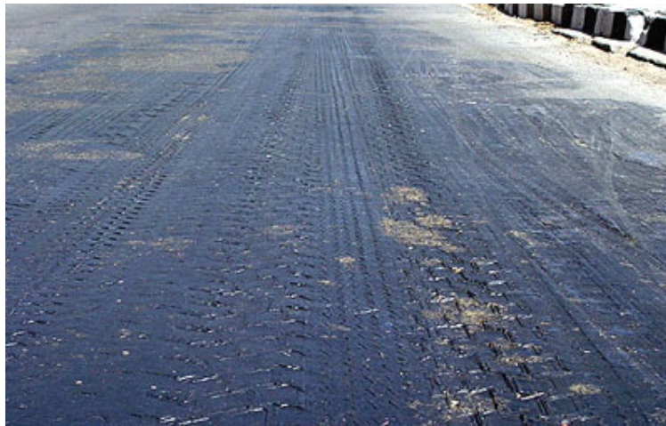
Photo: Bitumen Road (without plastics)
