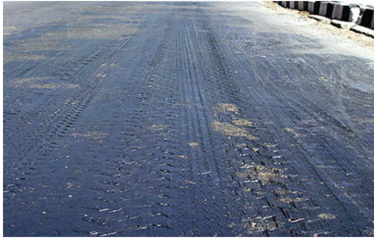
Photo: bitumen road (without plastics)
